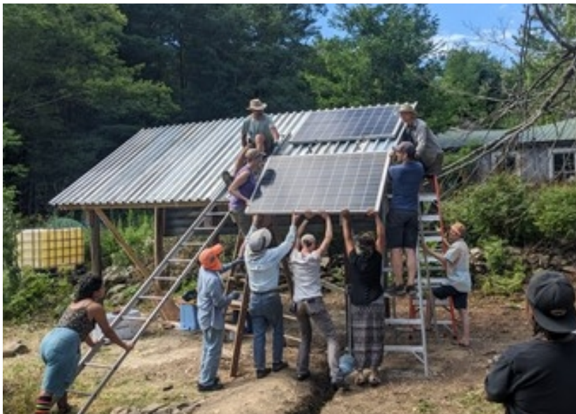
Installing solar panels at Serenity Solidarity.
