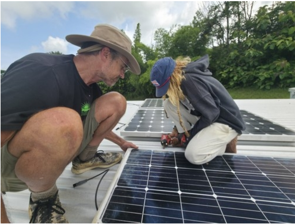
Tim and Ceilne install PV on the Forever Home for refrigeration, lighting and charging devices.
