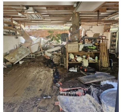
Flood damage at one of the houses that received our kits
