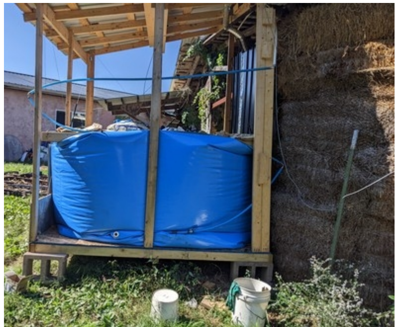
Our new, very large biogas storage bag is very helpful. All the gas we want, and stable pressure. Seymour (the digester) is nestled in the straw bales on the right.
