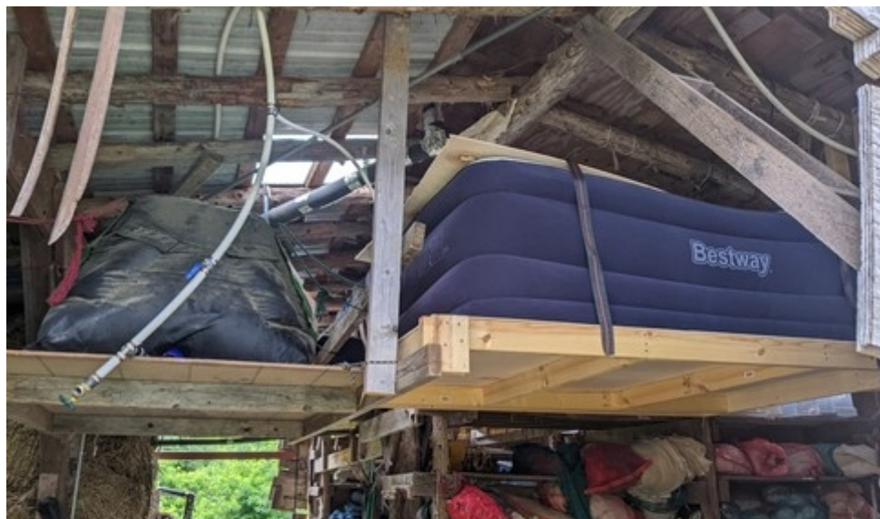
Biogas lofts in the barn. The commercial biogas bag on the left cost about $.43 cents/ liter of biogas storage. The air mattress on the right cost about $.03 cents/ liter of biogas storage. Smokers are not allowed to sleep on these air mattresses...
