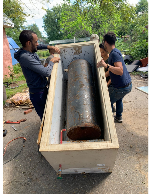
Building a batch collector at our 2023 training.
