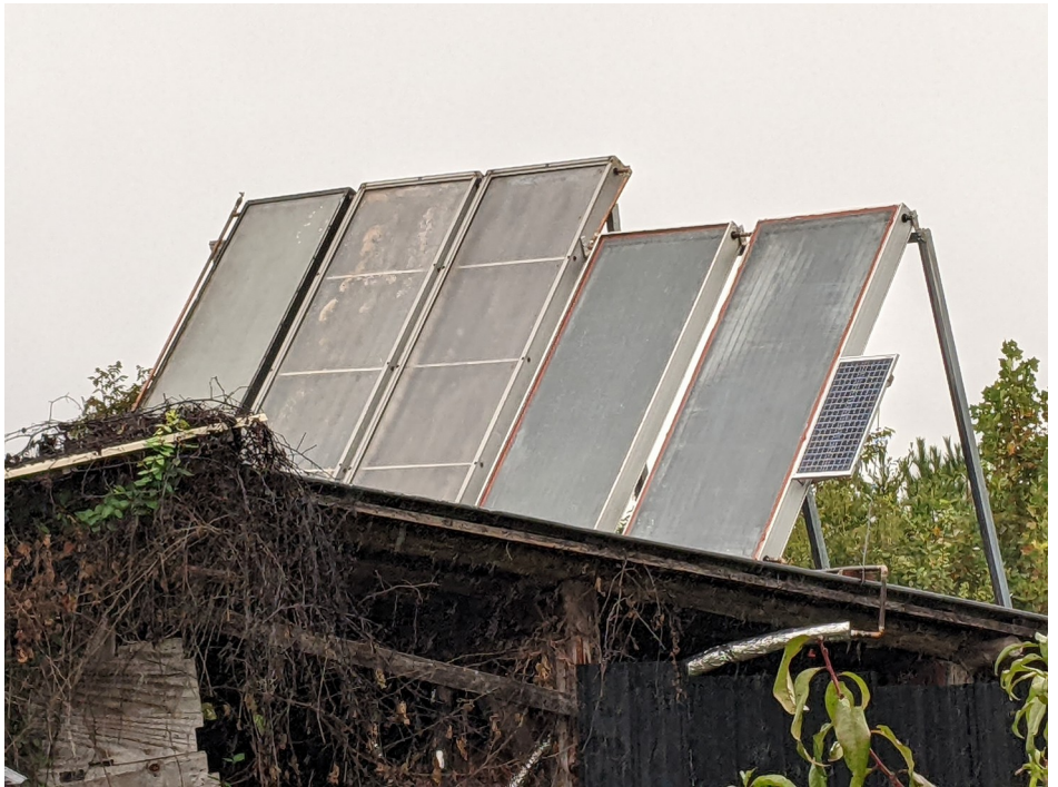
Solar thermal rack for our biogas digester, made from old thermal panels.
