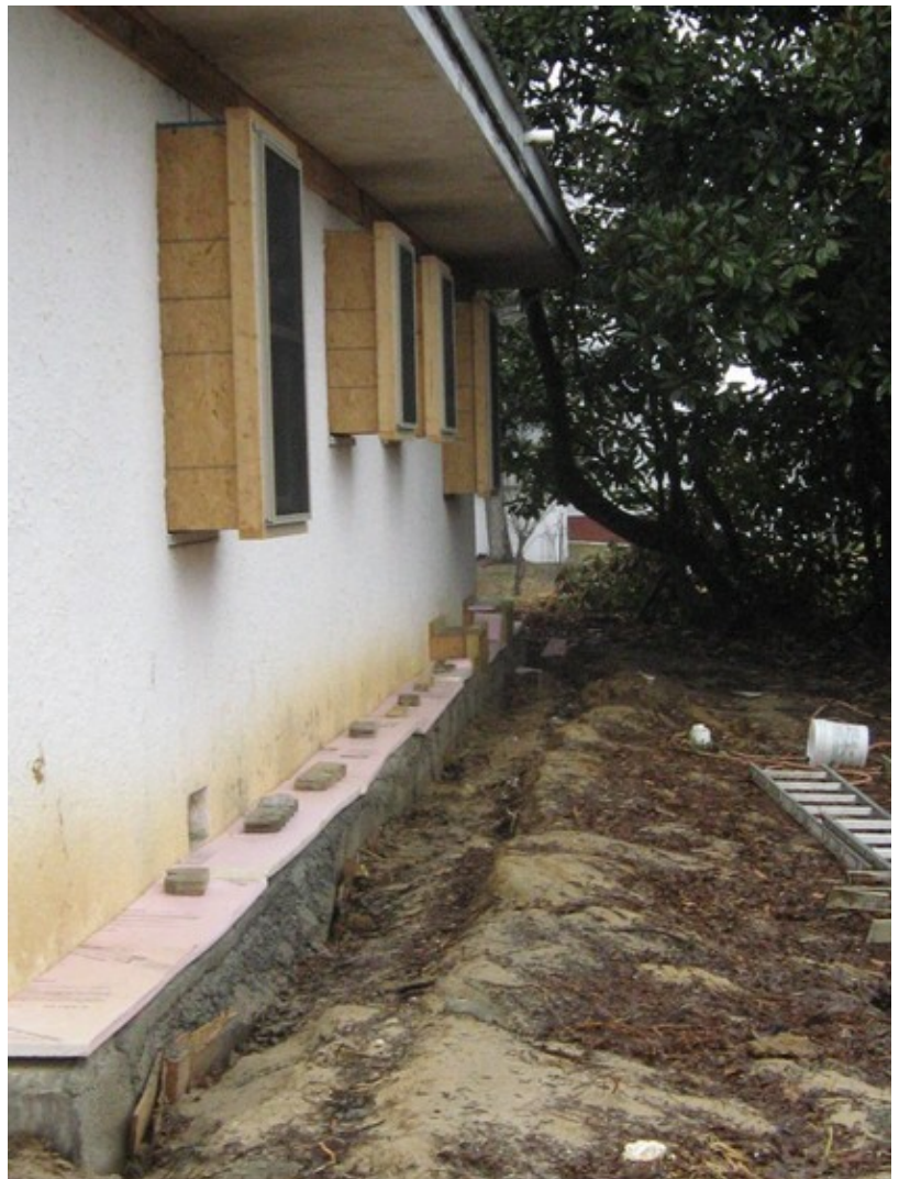
Magnolia House, windows boxed out and foundation ready for straw bales.
