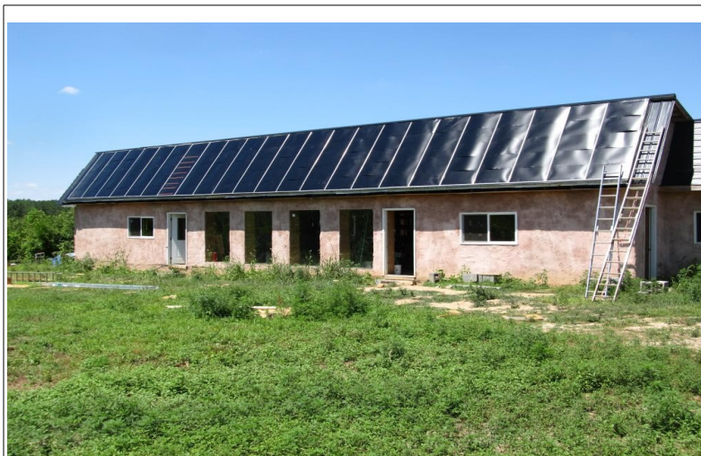
Solar Roof Sealed In, Ready for Glass and Ducts
