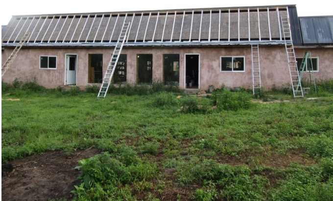
EarthHeart Solar Roof Construction Begins
