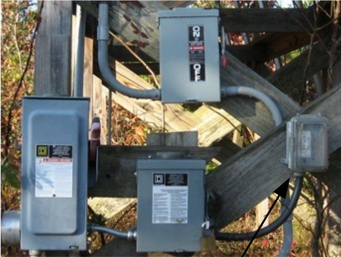
These are the control switches at our high-voltage PV rack. The timer on the right gets turned on once or twice a day to turn on the pump and pressurize the system.
