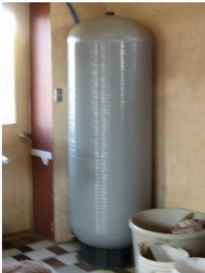
Most rural homes have a 20 - 30 gallon water storage tank, and rely on a pump that can run anytime of the day or night to supply water. Normal off-grid design relies on many thousands of dollars of electrical hardware to run conventional AC pumps at night. At LEF, we have 3 tanks like the one above, 120 gallons each. These tanks are not free, but overall system costs are much lower than conventional design.
