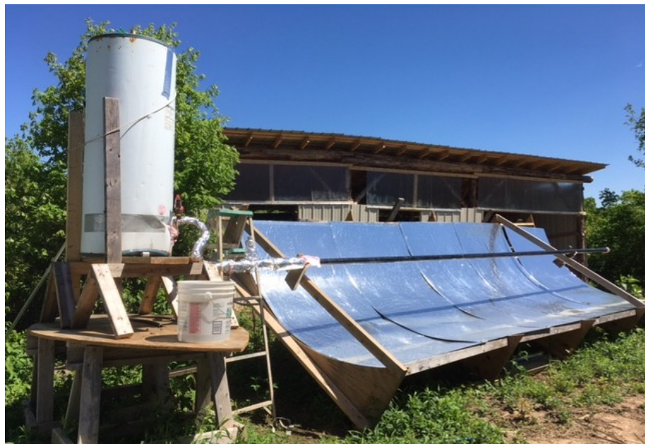
Solar boiler is operational, but not adequately effective (yet). New shop in the background.
