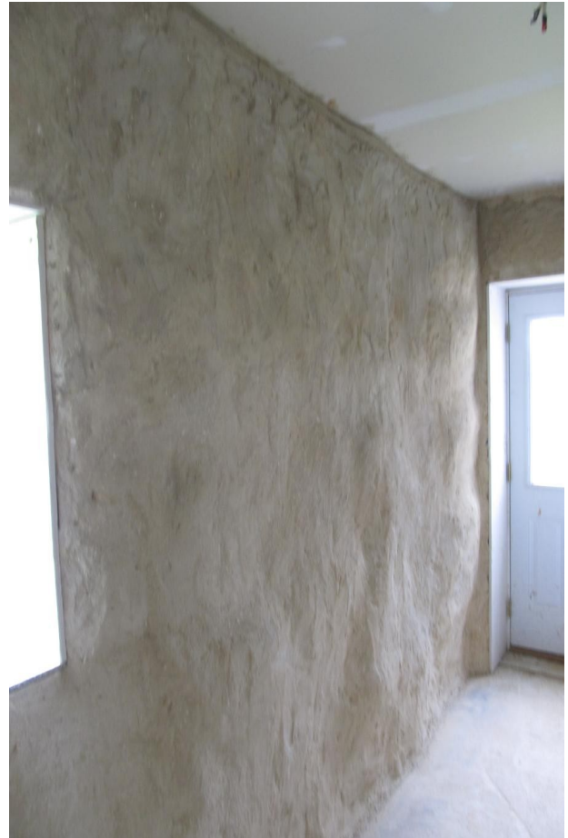
Finish Stucco Walls in EarthHeart
