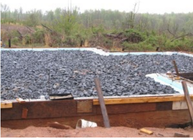
The foundation before pouring the slab.
