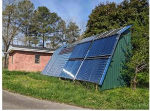
electric collectors. We are completing the thermal systems at this time. We are building a glycol based solar heat loop which will distribute heat through the old radiator system, originally used with a fuel oil boiler.
