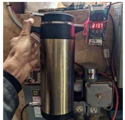
Load diverter (showing red numbers) and kettle for providing on-demand hot beverages.
