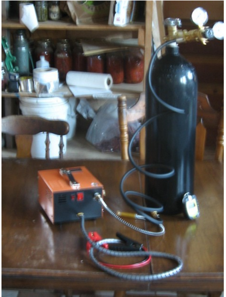
Biogas equipment to run a small tractor. Air rifle compressor, high pressure gas cylinder with regulator, hydrogen sulfide meter. We will have a biogas tractor running very soon, and this equipment cost less than $500.
