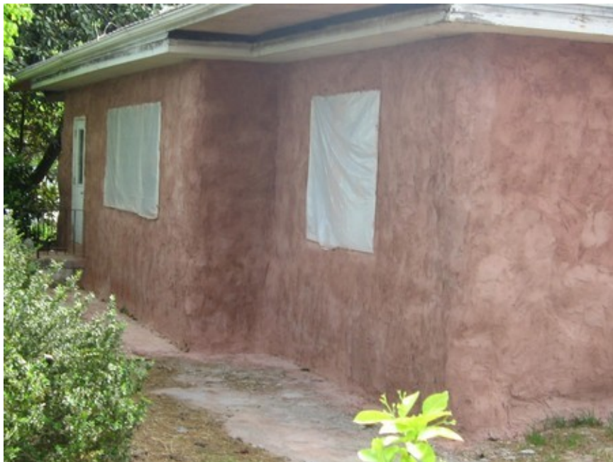
Magnolia, straw and stucco are done. Thanks to our hard-working crew!
