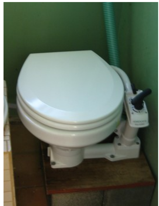
Biogas toilet with manual (pressurized) flush, uses a very small amount of water.
