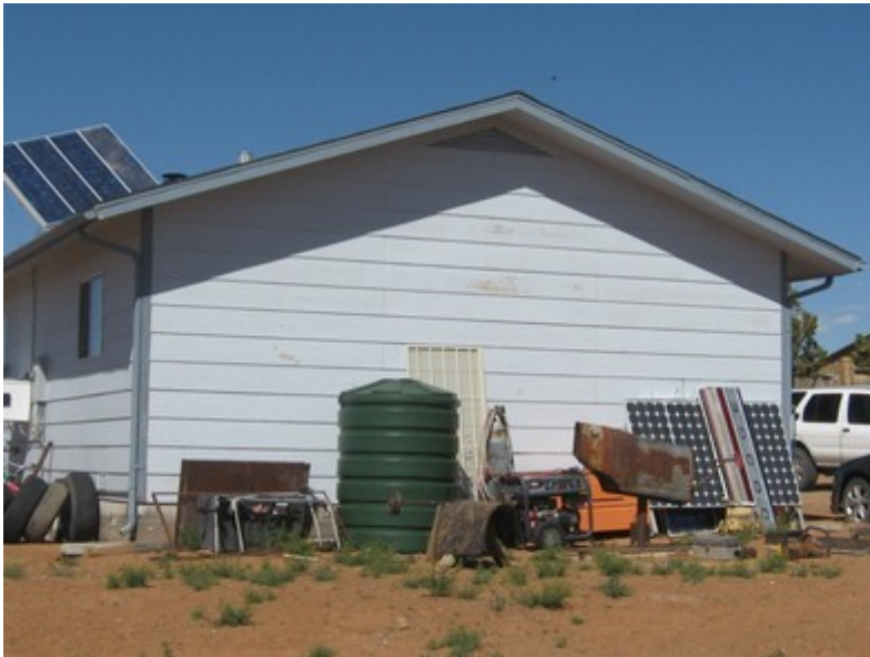
Site 2. The solar system with panels on the roof is non-operational, as is the one in the foreground. There are several sets of dead batteries. We utilized the solar panels and existing wiring, and tied our LELCS system into it.
