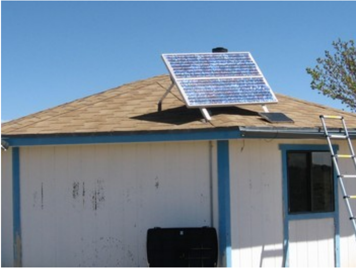
Site 4, family hogan with defunct $5,000 solar installation and dead batteries. We utilized the solar rack and internal electrical system, and swapped in our LELCS system to bypass the dead and corroded batteries.
