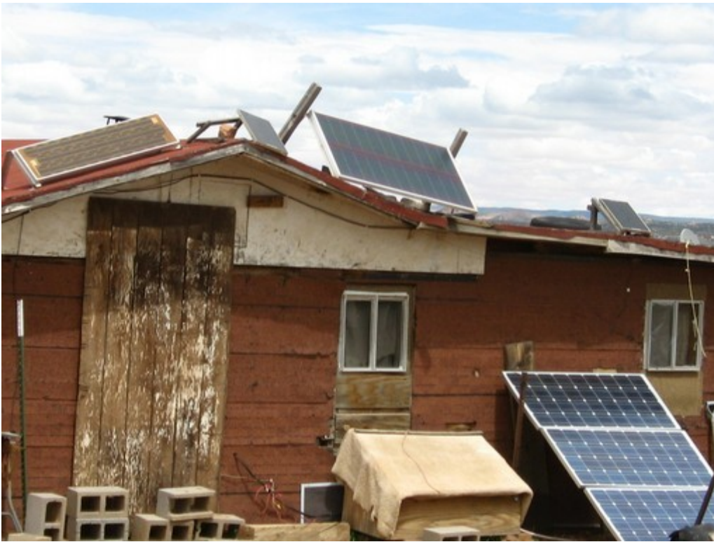
Site 7. There are several attempts at setting up solar electricity at this site. The beige box in the foreground is full of dead and corroded batteries. We were able to use the panel on the roof, and installed all new components from there.
