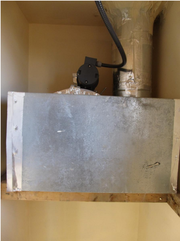
Daylight drive blower that heats the kitchen. We built a closet around the blower and put a diversion in the duct so we could blow hot air through the closet, which then functions as an industrial scale food drier.
