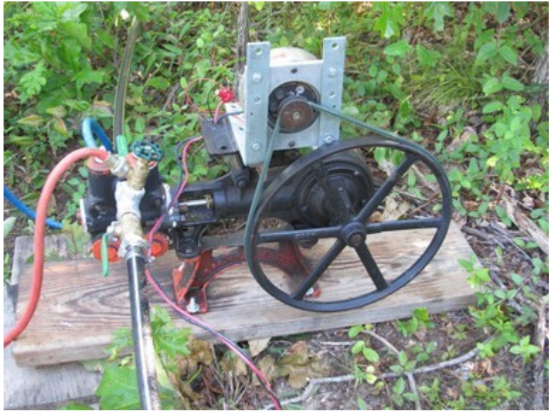
We love our 180 volt daylight drive because we can run powerful motors all over the community connected by small wires. But for remote use, low voltage daylight drive works too. This is a 24 volt daylight drive irrigation pump.
