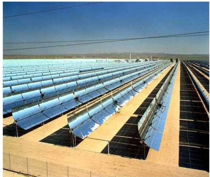
Industrial solar troughs, much more efficient than photovoltaic.
