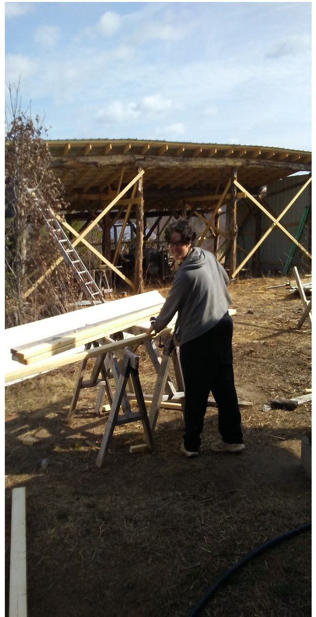
Deb building a duck house, new shop in the background!
